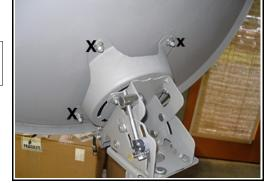
STEP 5 – Complete the assembly by installing the LNB head and fastening with either screws and nuts provided or using the clamp on the end of the LNB arm.
